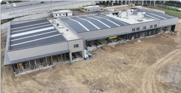
İETT / Atko Başakşehir Transport facility
